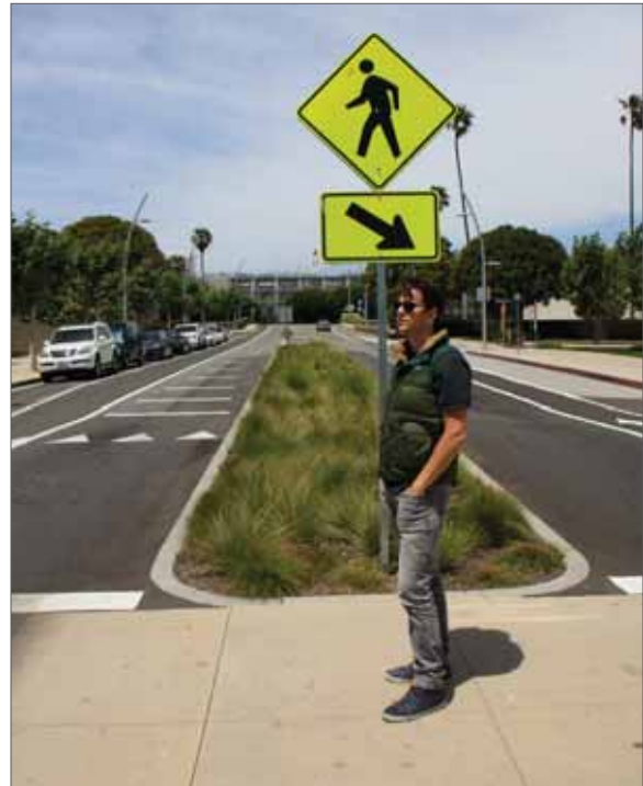
Mid-block pedestrian crossing with landscaped median, pedestrian refuge, and signage to alert drivers.
