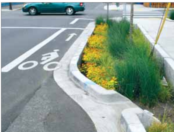
Stormwater run-off treatment.
