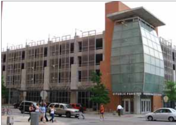
Public parking garage.
