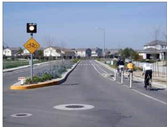
Striping of lanes, raised dividers, and painted buffers can help make bicycle lanes more visible.
