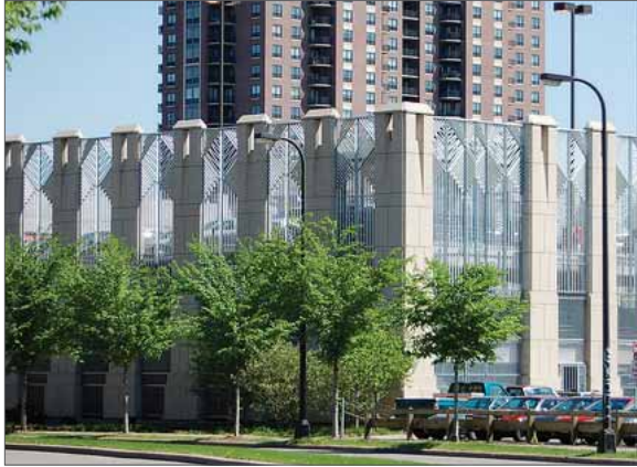
Screened parking garage.
