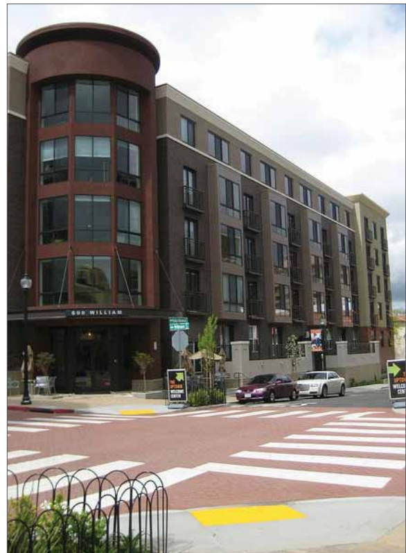
New sidewalks and crosswalks.
