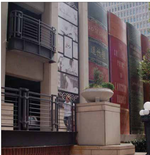
Screened parking garage.
