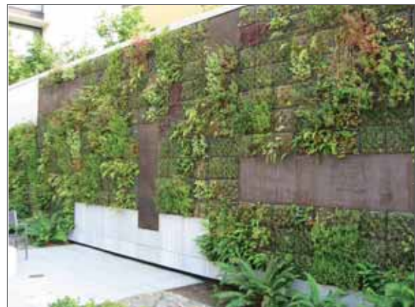
Green wall using graywater.
