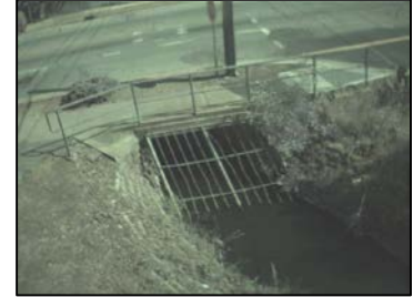
Photo 7a: Trash Rack in Morgan Hill
