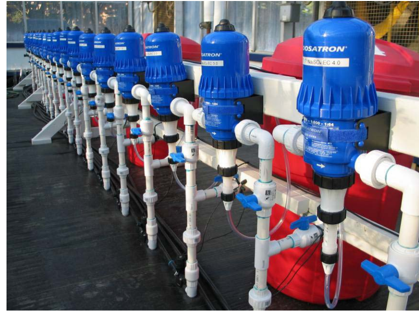
Figure 3. Injector system. Red cans intended for concentrate tanks were replaced with 8L bottles.
