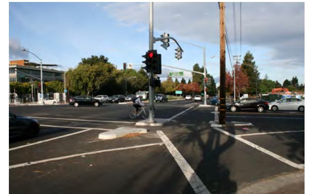
Removing the right-turn slip lanes would reduce vehicle turning speeds and provide additional pedestrian refuge space.
