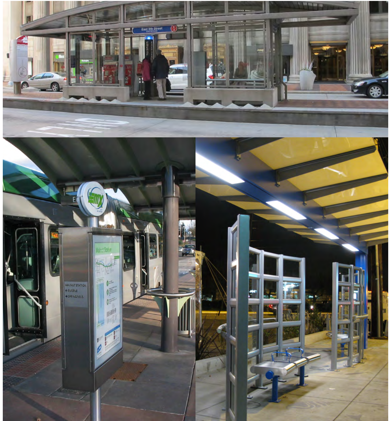
Transit stops will include shelter, lighting, benches, and other high-quality passenger amenities. Images from Flickr, ITDP (top); Flickr, Chris Phan (bottom L); Flickr Oran Viriyincy (bottom R)
