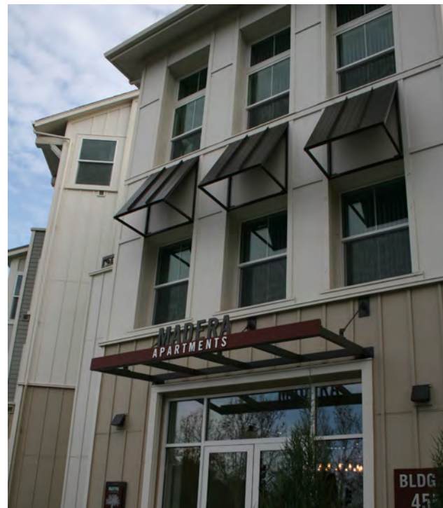
Additional mixed-use development near the Transit Center is being constructed and more is proposed.
