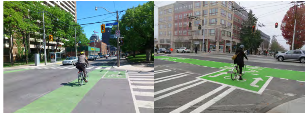
Two-stage turn boxes facilitate left turns across busy intersections. Images from Flickr, Payton Chung (left) and Flickr, Seattle DOP (right)
