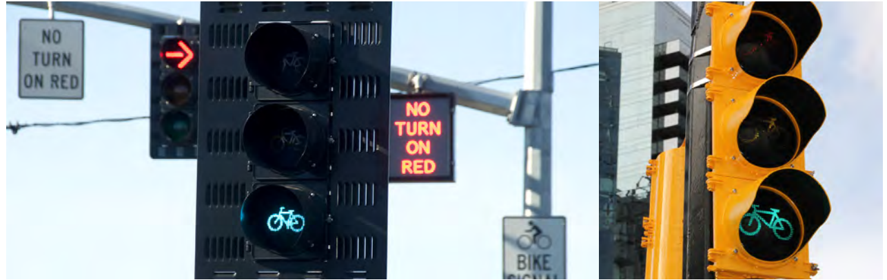
A dedicated signal phase for bicyclists will safely facilitate movements through intersections and mitigate right-turn conflicts. Images from Flickr, Oregon DOT (top); Flickr, Paul Krueger (right)
