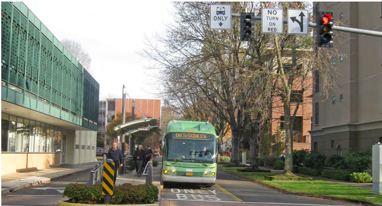
Dedicated signalization and signage at intersections will be used to control entry and exit into the transit lane. Image from Flickr, streetcar.press
