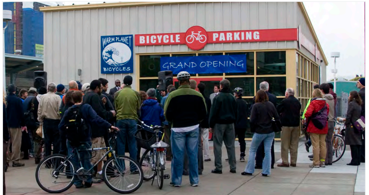
The existing station house building offers an opportunity for a staffed bike station, which can increase secure parking and provide an amenity to riders. One example is the bike station at 4th and King in San Francisco. Image from Flickr, ITDP
