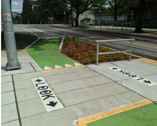
The bicycle lane buffer and pedestrian realm can include stormwater management features to reduce runoff and improve aesthetics.
