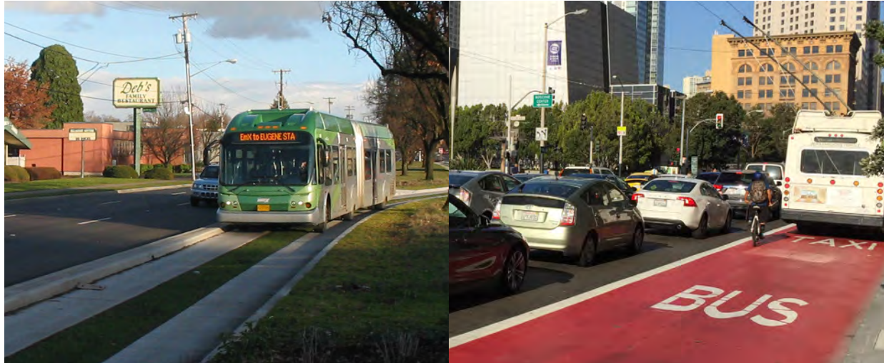
The median transit lane would be delineated by a combination of pavement markings and physical barriers.
