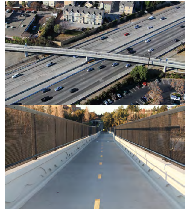
The recently completed Permanente Creek bridge over U.S. Route 101.
