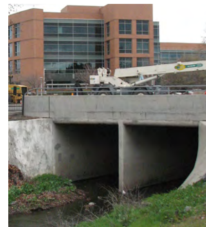
SLR CIPs include levee and floodwall improvements along lower Permanente Creek.
