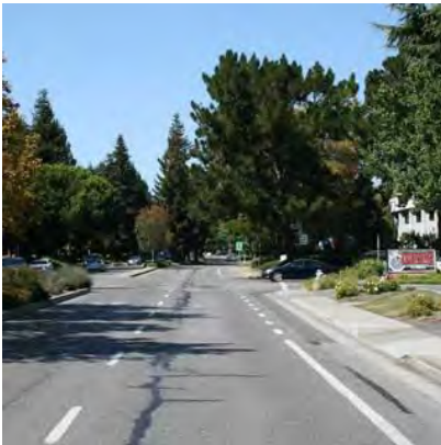
Shoreline Boulevard at Space Park Way, future Gateway Boulevard.
