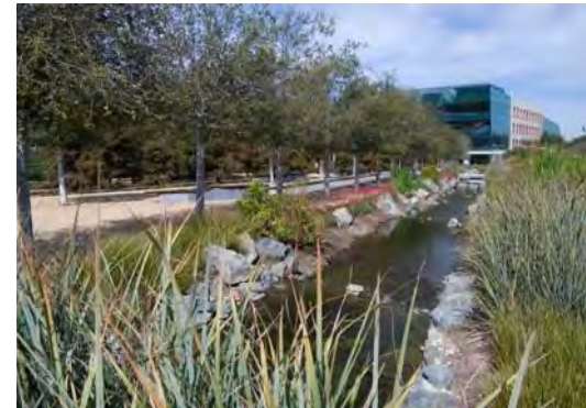
Example of sustainable landscaping, bioswales, and stormwater management integration.
