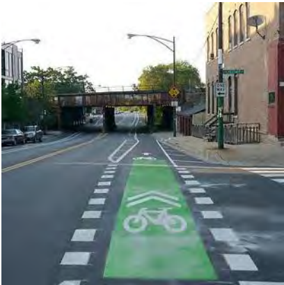
An example of highly visible bike lane markings.
