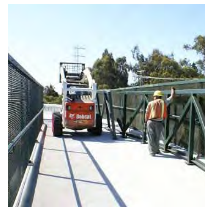
Permanente Creek Bridge construction.
