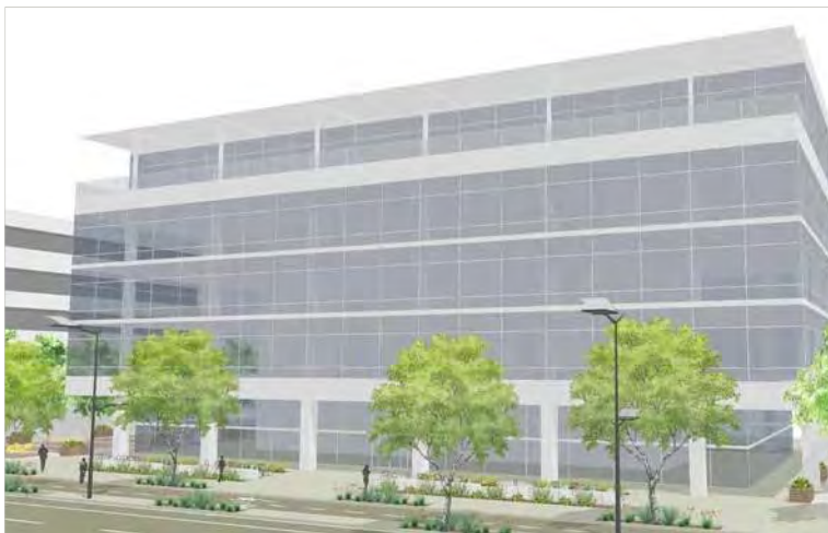
4d. Design of office buildings may have with simpler massing, including with relatively large unbroken façades, horizontally-oriented proportions, and repetitive fenestration.
