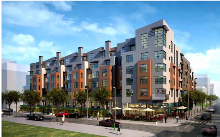
4c. Accentuate vertical massing of residential buildings may accentuate vertical massing with smaller scale vertically-oriented elements, emphasizing their height and access to light and views while providing a clearly residential building scale and character.
