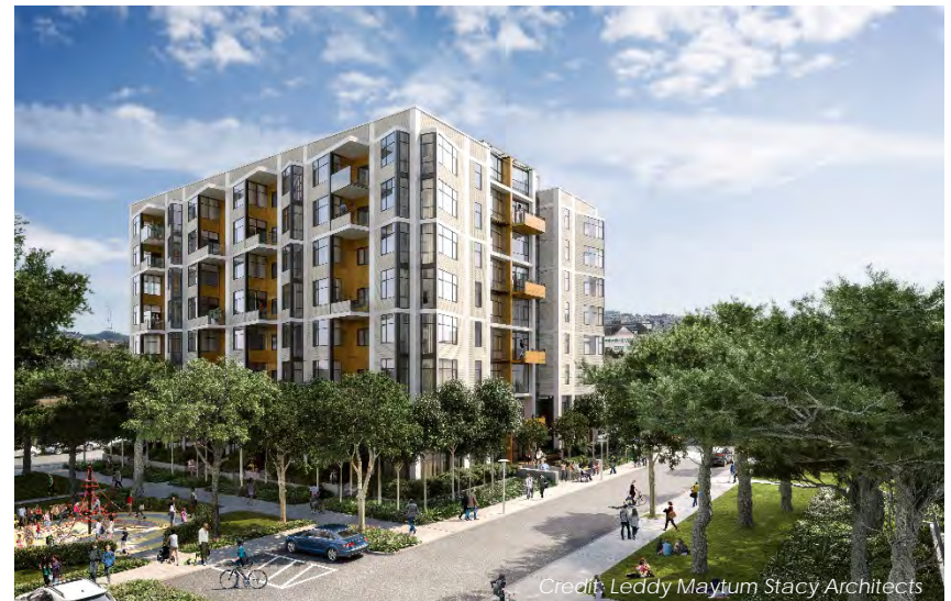
7m. Articulate residential building façades with smaller-scale increments than office building façades. Use windows, balconies, and bays for residential buildings to reflect the scale of residential rooms rather than open office floors. Taller residential buildings should have less building façade increments than mid-rise residential buildings.
