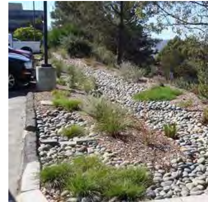
Bioswales provide stormwater capture and water filtration.
