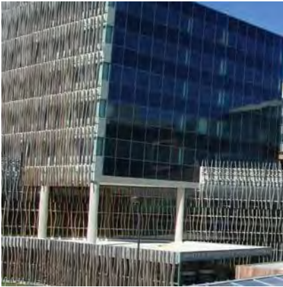
Windows are fronted by a 'brise soleil' or sunshade that makes the glass safe for birds.
