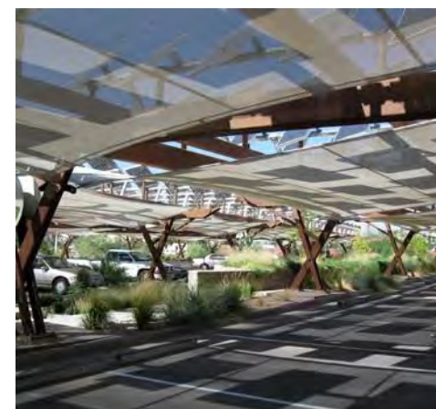
Overhead solar panels provide covered parking and contribute to local sustainability efforts.
