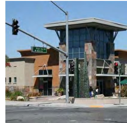
Intersection of Pear Avenue and Shoreline Boulevard.
