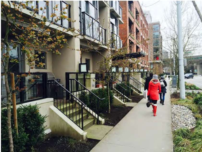
7ne. Integrate balconies with a building's massing to generate simple, urban facades. Balconies should employ high-quality materials, design and detailing, including on their underside.
