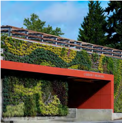
An example of an attractive parking entry.
