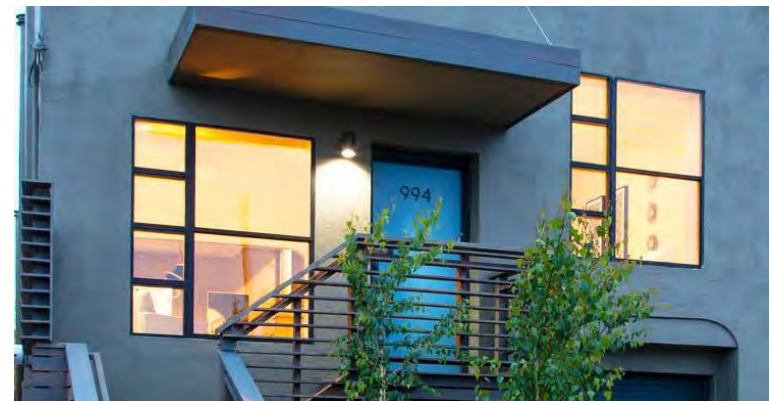
5l. Shelter Residential entries should be sheltered from the rain and wind and include an entry light.
