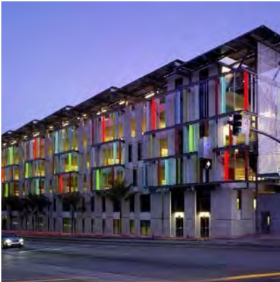
An example of a lined parking structure.
