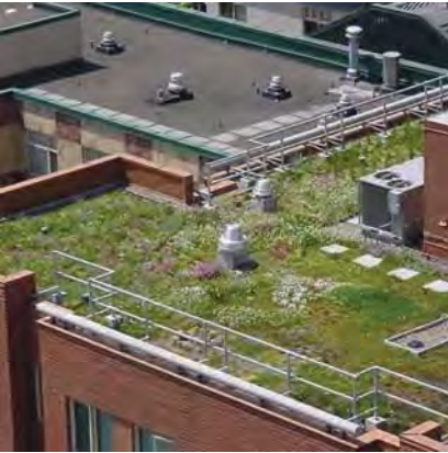
Vegetated roofs cool buildings and provide on-site stormwater filtration.
