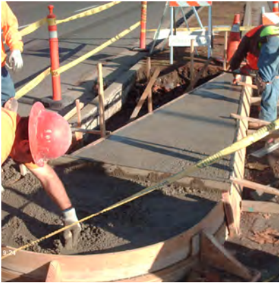
Sidewalk reconstruction in Mountain View.
