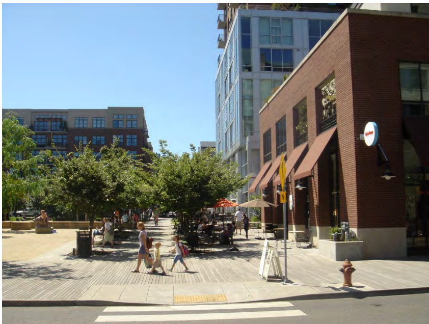
7op. Use visual and physical design cues within a building's design and entries to emphasize pedestrian and bicycle connections to public and natural spaces such as parks, greenways, trails, and open space.
