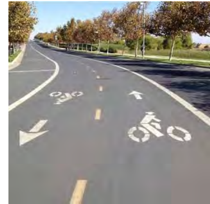
An example of a two-way cycle track next to a bus only lane.
