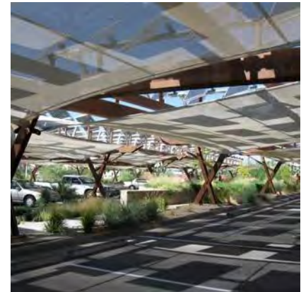
An example of a solar-shaded
