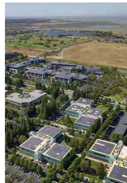
Solar panels on North Bayshore office buildings.
