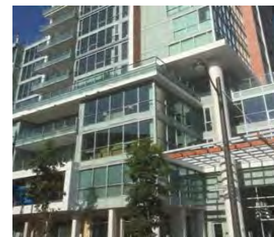
High-intensity residential buildings mark prominent locations.
