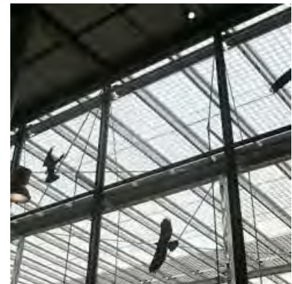
An example of external screens and stickers of birds of prey silhouettes
