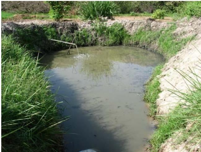
Figure 2 Loading narrow well with raw wastewater (Gaye and Niang, 2010)
