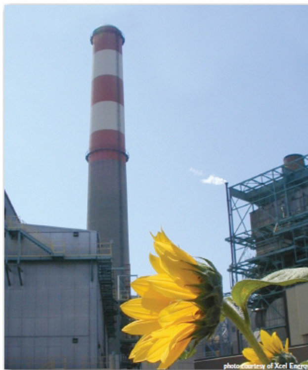
Figure 1 Cherokee Station (Photo credit: Xcel Energy)
