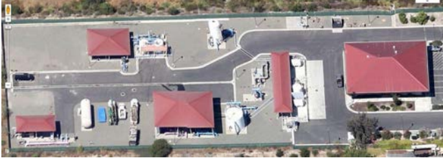
Figure 2 LVLWTF site (Photo credit: CDM Smith 2011)
