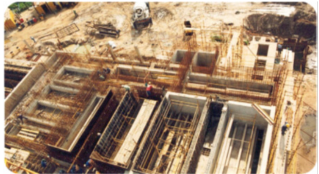
Figure 1 Construction of the Durban Wastewater Recycling Plant (Photo credit: Ethekeweni Metro Water Services)
