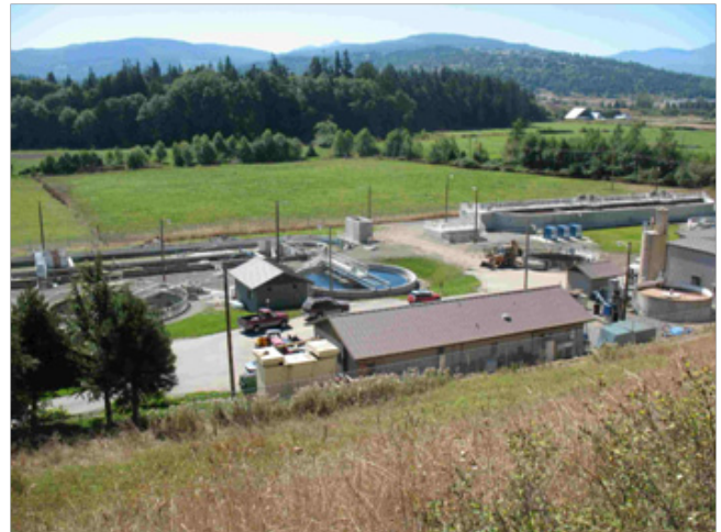
Figure 2 Sequim Water Reclamation Facility expansion (Photo credit: Gray & Osborne, Inc.)
