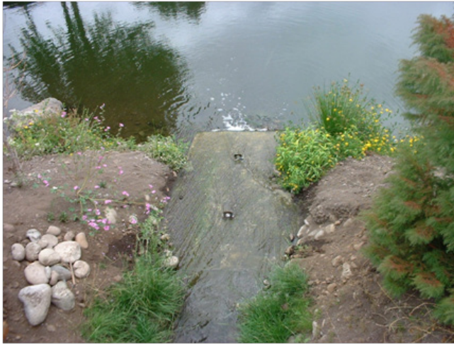
Figure 1 Introduction of reclaimed water to Bell Creek (Photo credit: Gray & Osborne, Inc.)
