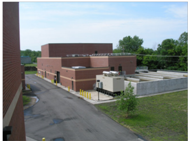
Figure 5-21 Mankato Water Reclamation Facility
