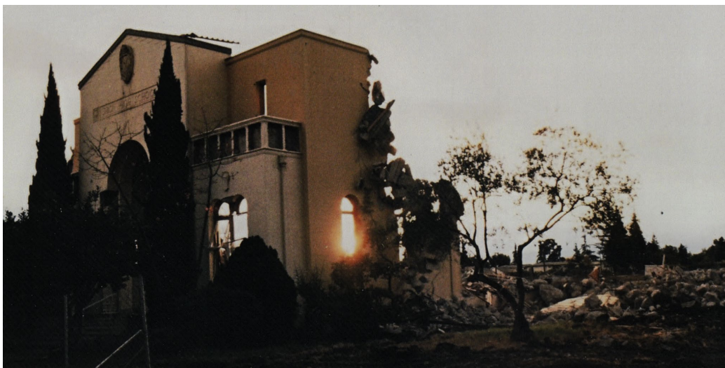
Demolition of Mountain View High School, 1987
