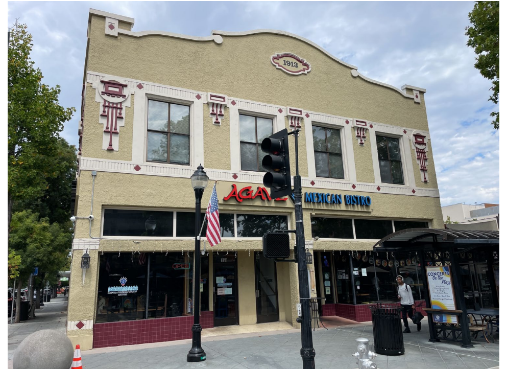
Jurian Building on Castro Street, 2022. Source: Page & Turnbull.
