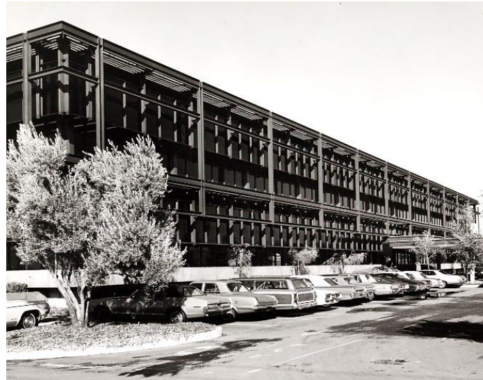
Fairchild Semiconductor aka the "Rusty Bucket." Demolished in 1993. Source: Mountain View Public Library.
