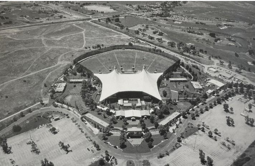
Shoreline Amphitheatre under construction c. 1980s. Source: Robert Weaver.
