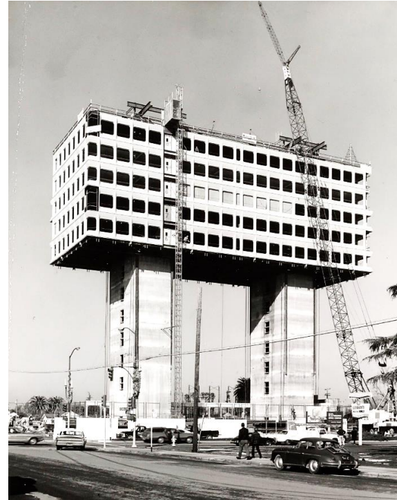
The IED Building under construction in 1970. Source: Mountain View Public Library.
